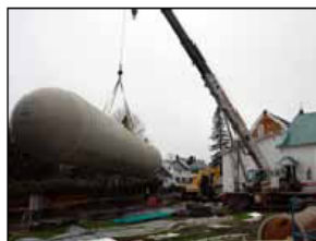
A 2000 gallon Water Tank Needed to Be Buried
