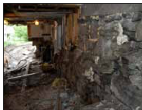
Foundation in June
