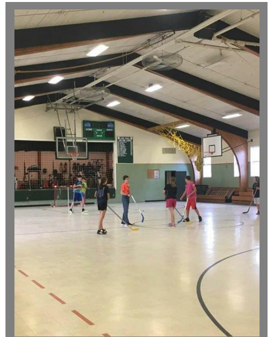
Ready for an upgrade.
